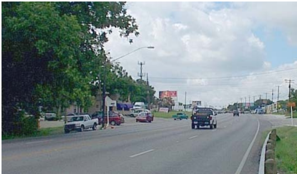
South Congress Avenue near Williamson Creek facing south. The lack of curbs and gutters along this segment are more akin to a rural highway rather than a major arterial road in a developed metropolitan area.
