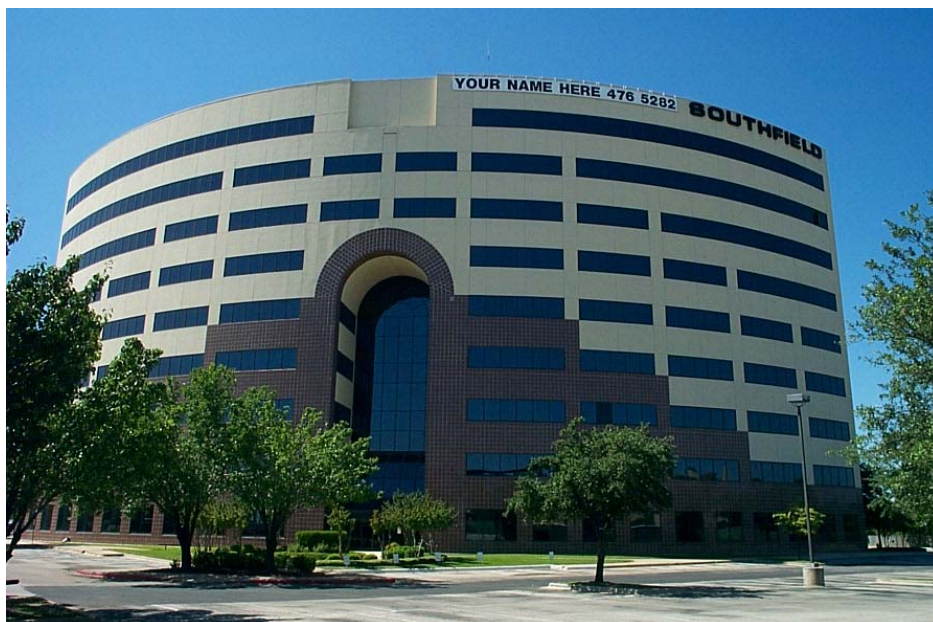
The Southfield building located at the northwest corner of Ben White Boulevard and Interstate Highway 35 is an example of the type of building desired along the eastbound frontage road.
