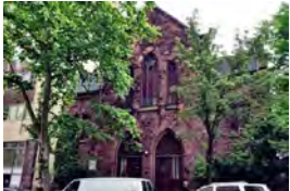
St. Peter's Church New York, NY Consulted on the conversion of a historic church into 36 ultra-luxury condominiums in Brooklyn Heights. Sold out in 6 months
