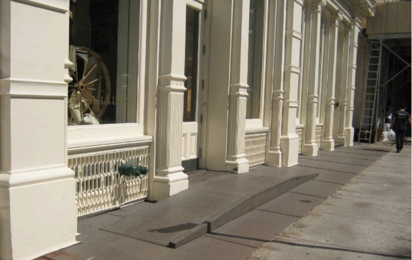
Above: Ramps and chair lifts can provide access while preserving historic character.
