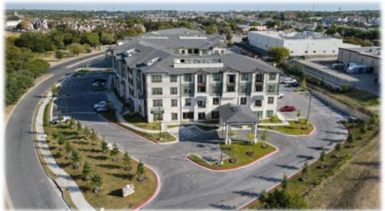
Heritage Estates at Wells Branch (174-unit senior-living development in Austin, Texas at 14011 Owen-Tech Blvd.). Heritage Estates at Wells Branch was completed in the last quarter of 2022 is over 50% occupied as of March 2023.
