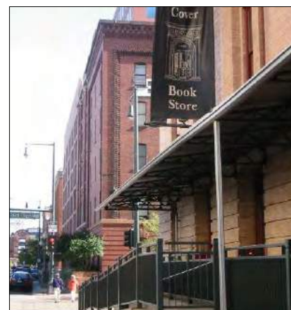
Figure 5-2: Example of an ADA ramp with shade structure
