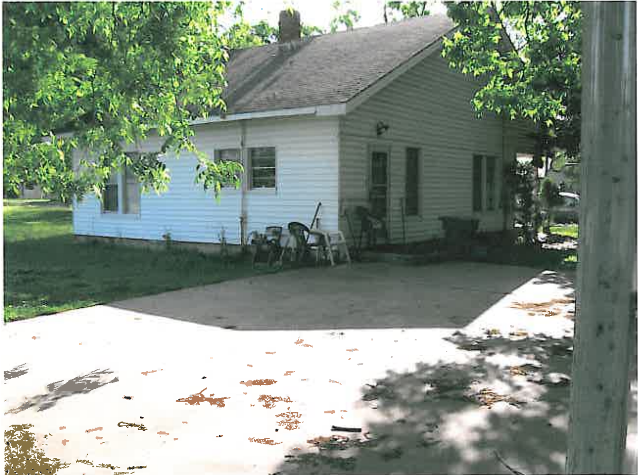
Photo 2 View of converted garage structure at 1126 Tillery
