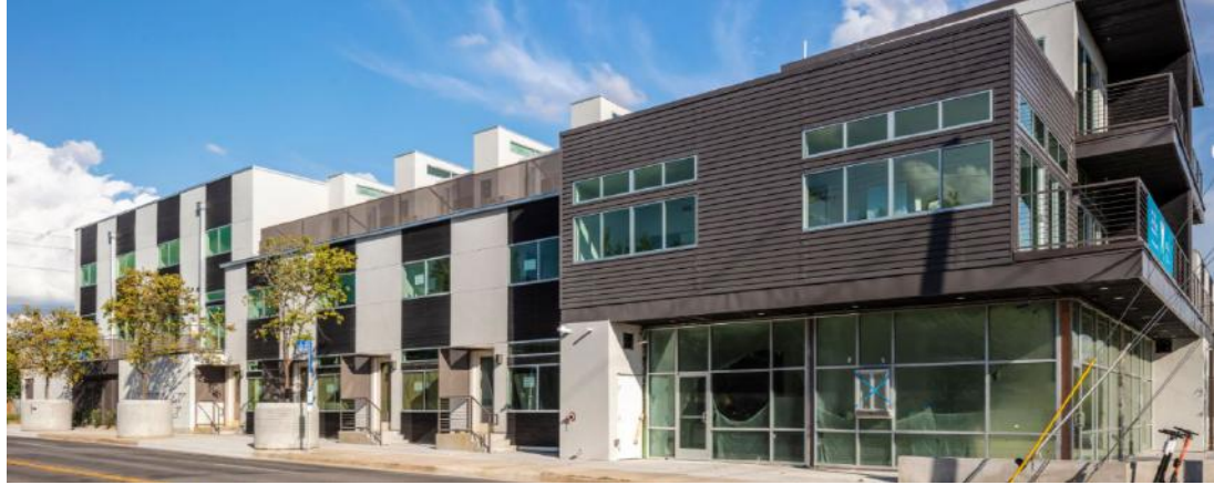
Permanent Modular housing in downtown Austin
