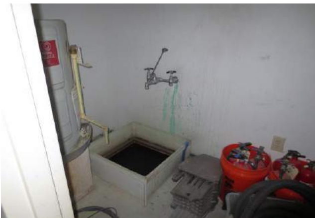
Photo 41 View of the janitorial floor sink within the on-site MSC building
