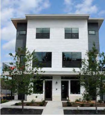
AGAVE LOFTS AT TOWN CREEK NEW BRAUNFELS, TEXAS $2,200,000
