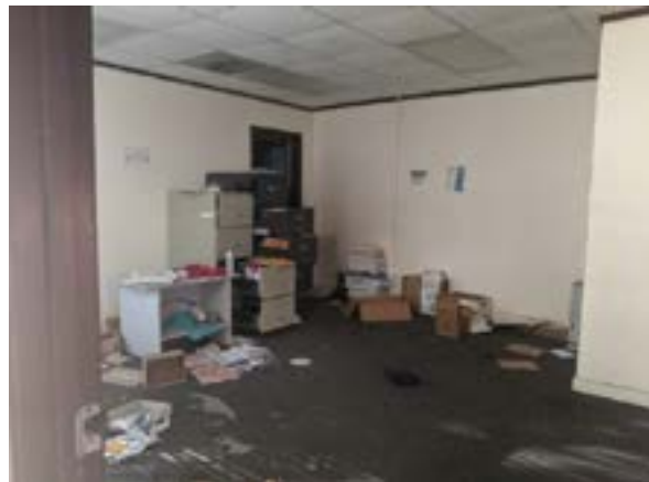
Photo 18 Interior view of the on-site building
