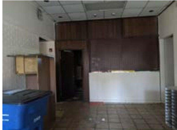
Photo 14 Interior view of the on-site building
