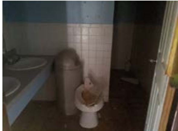
Photo 16 Interior view of the on-site building
