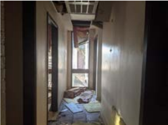
Photo 15 Interior view of the on-site building
