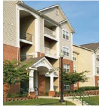
WOODMONT CROSSING APARTMENTS 2327 Good Hope Road SE Washington, DC 20020 176 units
