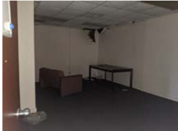
Photo 22 Interior view of the on-site building
