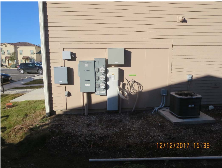
EAST MEADOWS BLOCK C BUILDING 28 2017 12-12.1 Photo #118
