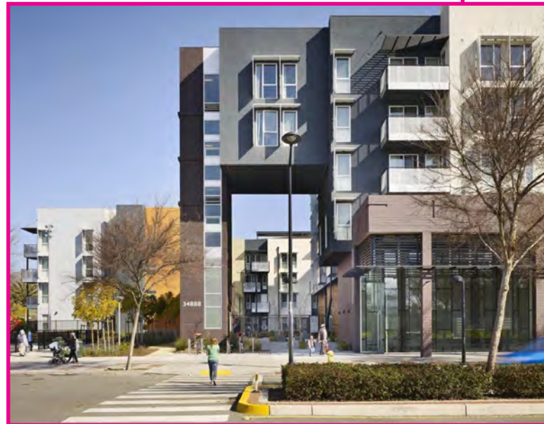
Figure 4-2: Station Center, Union City, CA: This master-planned district leveraged the collective financial investments to support development of Station Center, a green and an innovative affordable housing community with commercial space that provides 157 homes for low-income working families or individuals.
