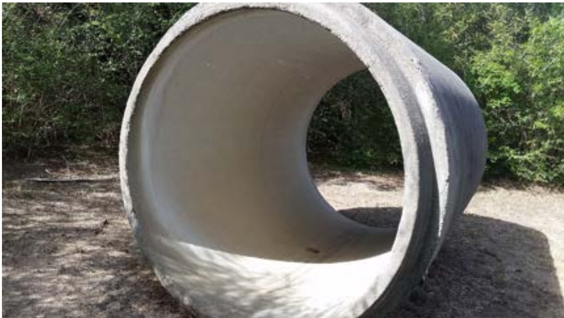
No. 6 – Photograph of the concrete culvert on Subject Property.
