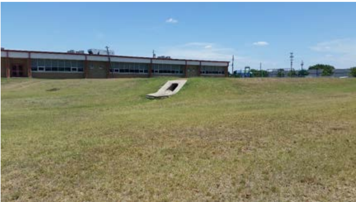
No. 14 – Photograph of adjoining property, , Noman Elementary School Infiltration Basin storm water structure.
