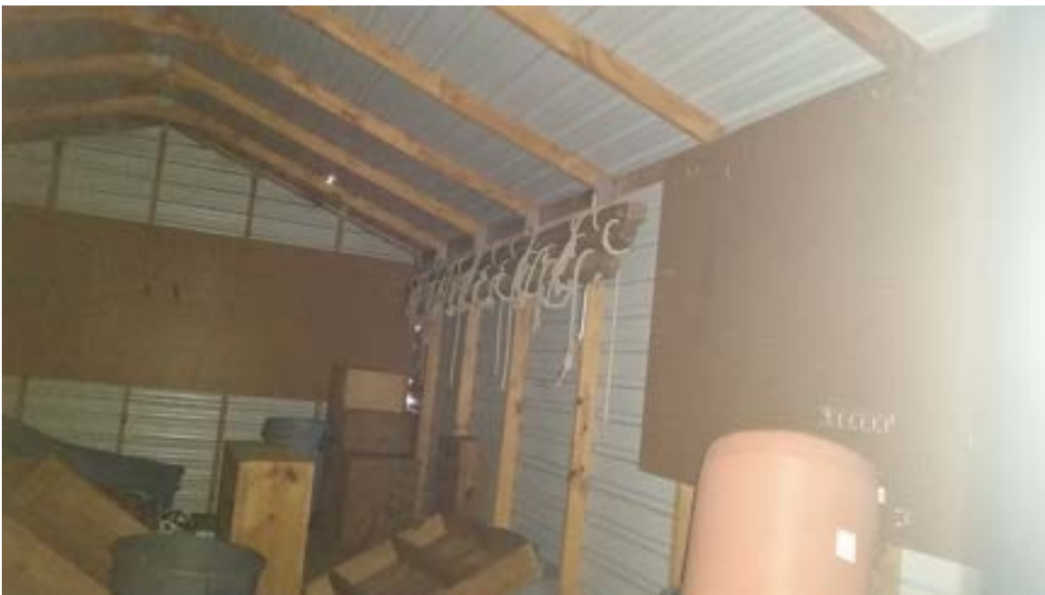
No. 10 – Photograph of inside of the storage building.
