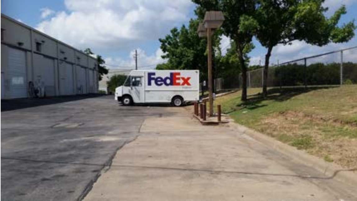
No. 21 – Photograph of the former fuel dispensing area at Fed Ex.
