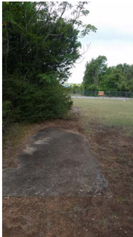
No. 12 – Photograph of the concrete slab on the Subject Property.
