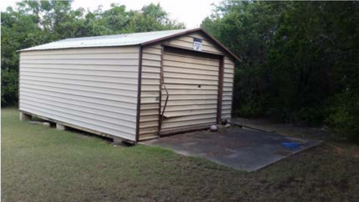
No. 9 – Photograph of the Storage Building.
