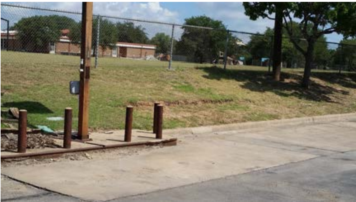
No. 20 – Photograph of northeast adjoining property, former fuel dispensing area at Fed Ex.
