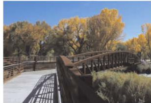
North Animas River Pedestrian Bridge- Aztec, NM
