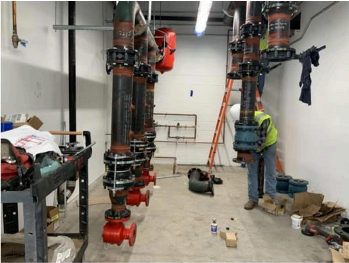
Central Utility Plant (CUP): Chilled water to pump connections in progress.
