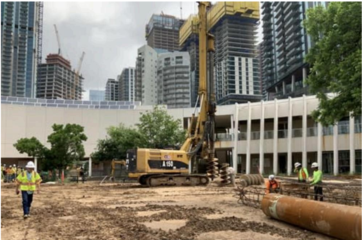
Zocalo: Foundation work: Shade structure drilled piers underway.
