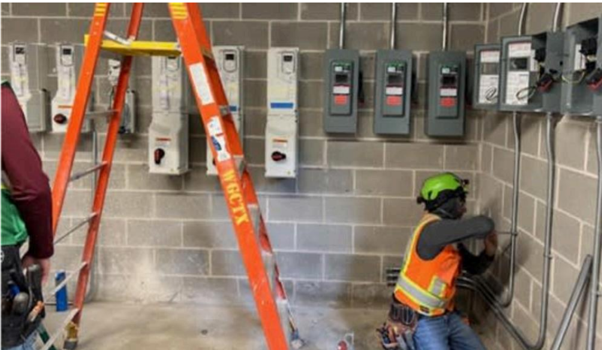
Central Utility Plant (CUP): Electrical connections in progress.
