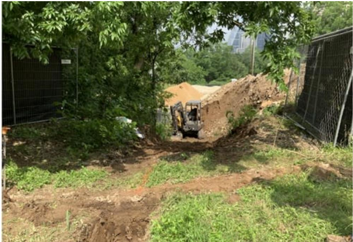
Site: North stormwater outfall trenched and backfilled.
