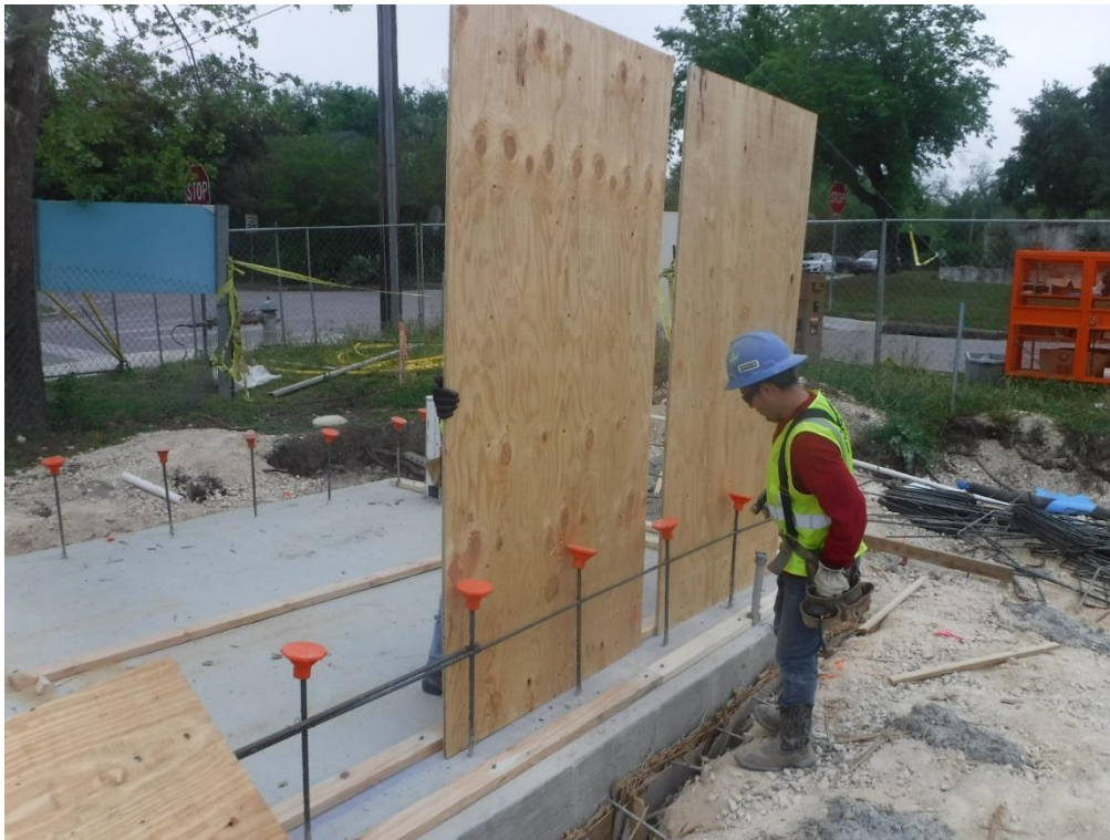
Installation of forms for concrete walls at bathhouse
