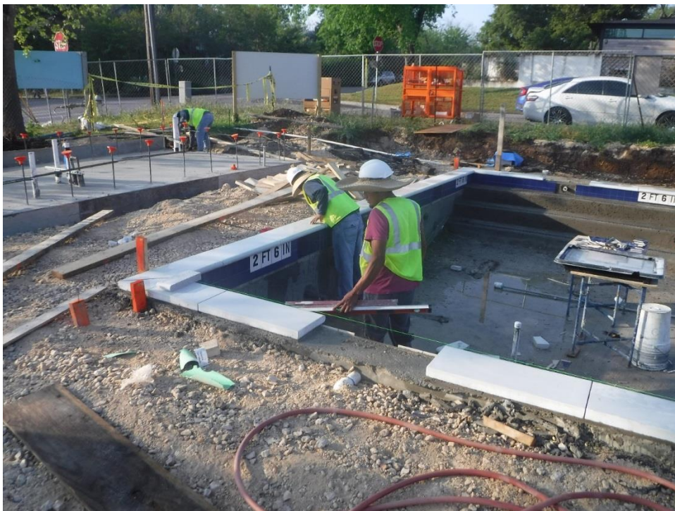
Coping and tile installations at activity pool. Restroom foundation slab in background
