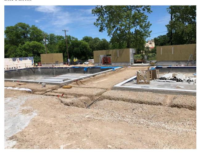
Completed building forms with insulation attached, prepared for limestone finish. Pool coping completed along with tile at pool water line.
