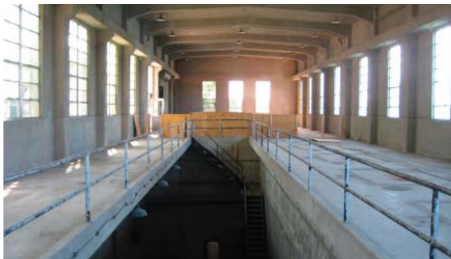
Building A: Upper level voids.
