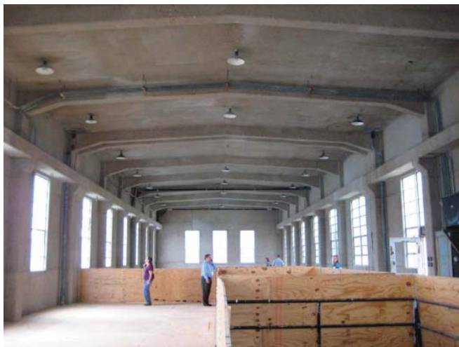
Building A: Ground Level Interior Space
