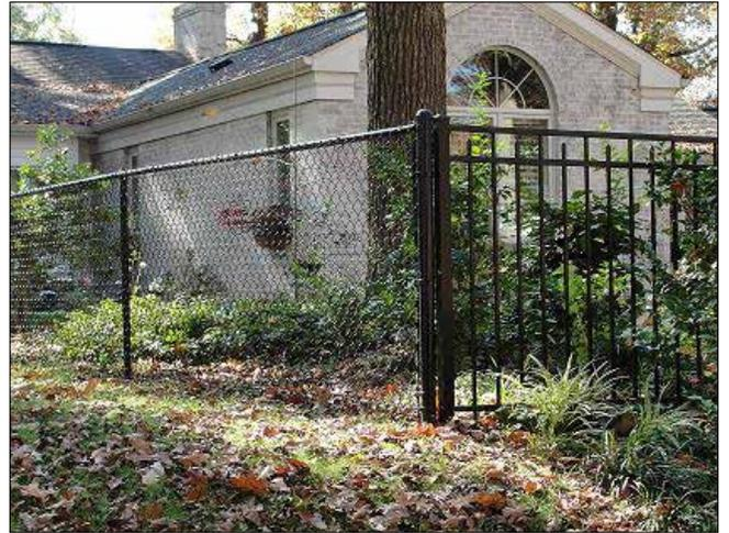
Figure 18. Black chain link is less expensive than steel picket fence and can be used for areas of low visibility.. (Atlas Fence)
