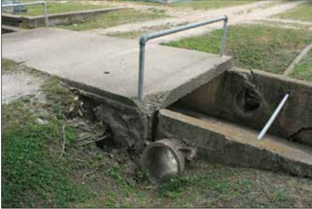
Figure 185. Soil washout along the side of the channel (John Milner Associates)
