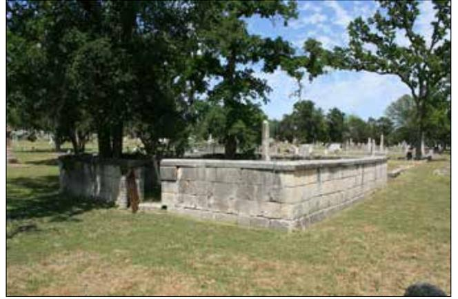
*Figure 164. Limestone masonry wall surrounding a family plot in Section 4 (John Milner Associates)*
