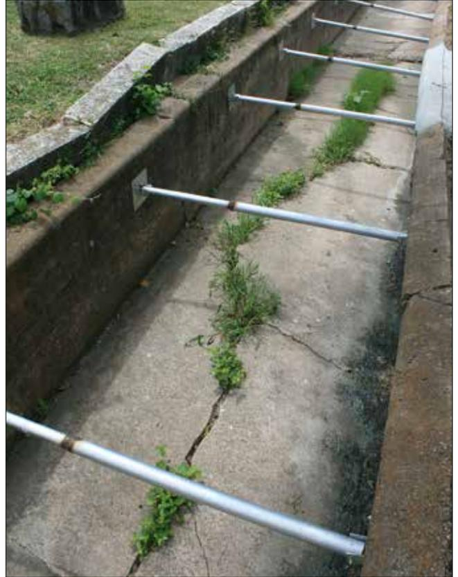
Figure 182. Cracked channel bottom (John Milner Associates)
