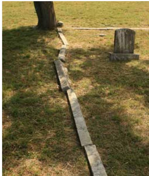
Figure 162. (left) Severely damaged limestone curb, probably due to mowers; (right) displaced curbing (John Milner Associates)
