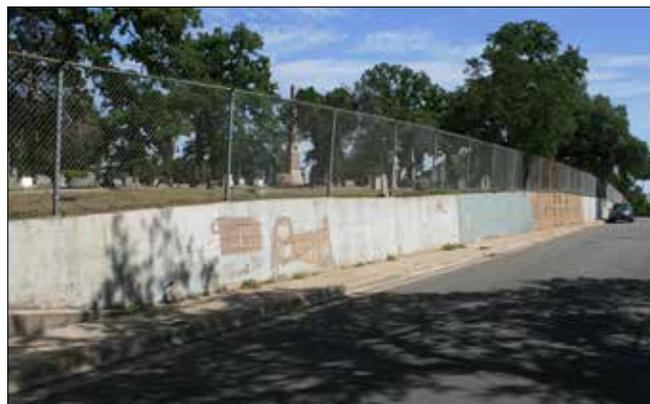
Figure 198. A concrete retaining wall along the southwest corner (John Milner Associates)
