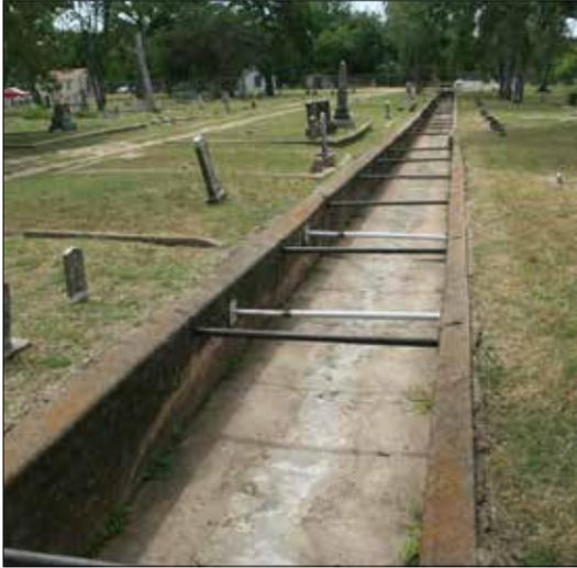
*Figure 179. The concrete drainage channel that bisects the cemetery (John Milner Associates)*
