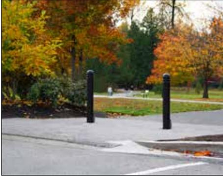
Figure 220. Removable steel bollards
