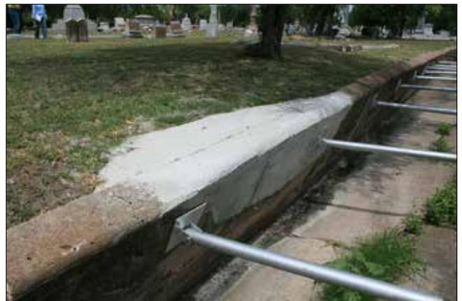
Figure 184. Recent repair of a collapsed wall segment (John Milner Associates)
