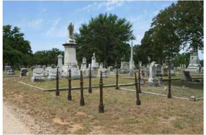
Figure 167. Missing fencing (John Milner Associates)
