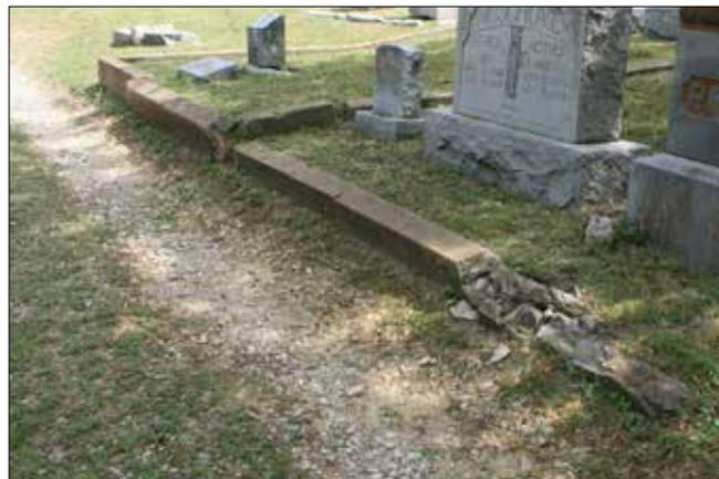
Figure 73. Eroded road beds are causing adjacent features to lean and break, as is visible in the curbing here. (John Milner Associates)
