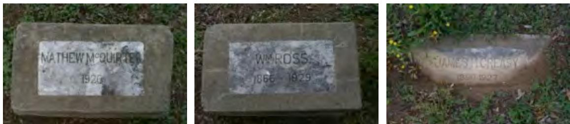
Figure PL-5. Stone markers in concrete; Creasy marker (right) is sunken and shows mower damage.
