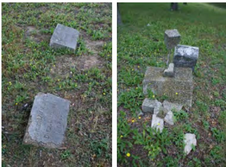
Figure PL-11. (Left) mower damage; (right) broken concrete cross.
