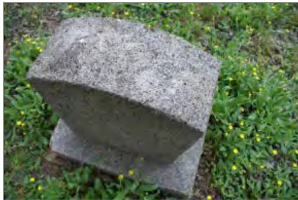
Figure PL-4. Concrete grave marker with distinctive mica aggregate.
