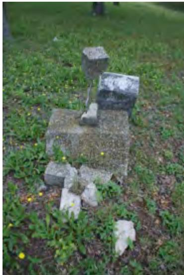
Figure PL-11. (Left) mower damage; (right) broken concrete cross.
