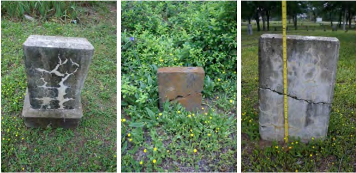
*Figure PL-12. (Left to right) Repaired cracks; cracked marker; cracked marker with visible repairs.*
