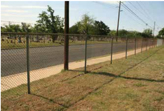
Figure 288. A chain link fence topped with barbed wire surrounds the cemetery. (John Milner Associates)
