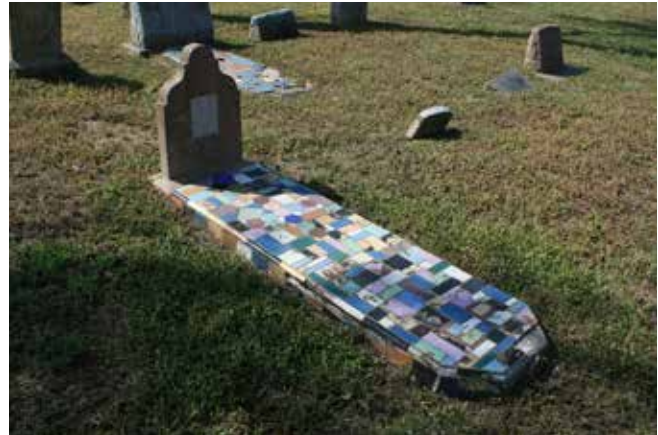
Figure 278. A concrete plot covering set with decorative tiles (John Milner Associates)
