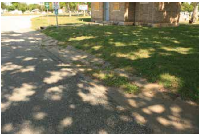
Figure 283. Concrete gutter along the cemetery entrance drive (John Milner Associates)
