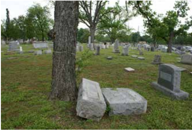
Figure 260. Marker displaced by a nearby tree trunk (McDoux Preservation)
