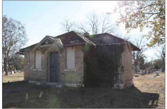
Figure 227. Gate house, Oakwood Cemetery Annex, before restoration (Dale Flatt)
