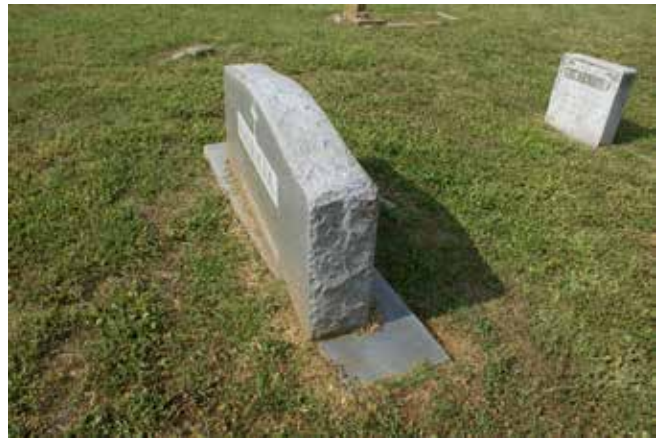
Figure 270. Displaced marker, possibly by contact with a mower (McDoux Preservation)
