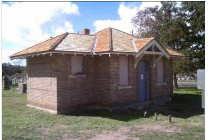
Figure 228. Gate house, Oakwood Cemetery Annex, during restoration (City of Austin)
