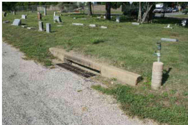
Figure 284. Drop inlet with curb; an irrigation riser embedded in concrete stands adjacent. (John Milner Associates)
