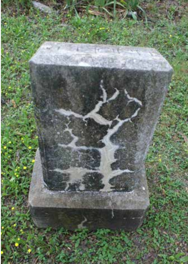
Figure 327. Repaired cracks (McDoux Preservation)
