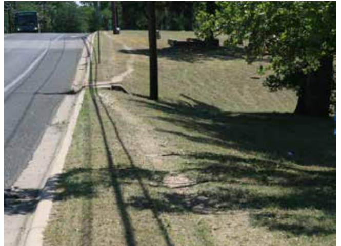
Figure 302. Social trail on cemetery grounds along Springdale Road (John Milner Associates)
