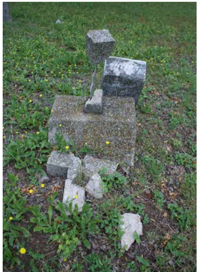
Figure 322. Broken concrete cross (McDoux Preservation)
