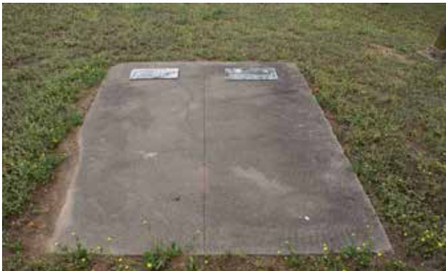
Figure 330. Family plot covered with a poured concrete slab (McDoux Preservation)
