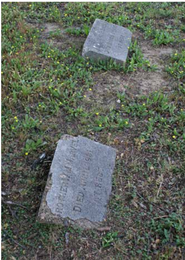
Figure 321. Mower damage (McDoux Preservation)
