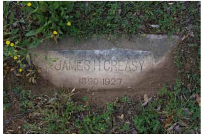
Figure 320. Stone marker in concrete; the marker is sunken and shows mower damage (McDoux Preservation)
