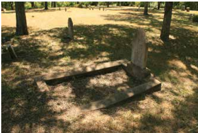
Figure 334. The curb surrounding this individual burial is slightly sunken at one corner (John Milner Associates)
