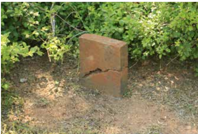
Figure 329. Cracked marker (John Milner Associates)
