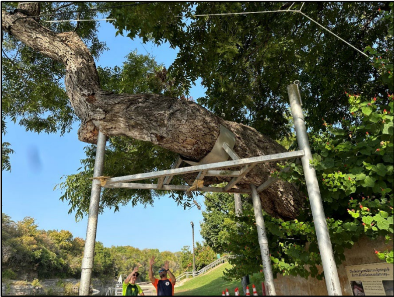
Image 1: View from the sidewalk under the pecan. Previously installed props and a soft “cabling” system pictured.
