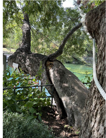
Image 5. Concrete filled cavity leaning over guardrail and sidewalk below. Rebar and expanding foam was also observed.
