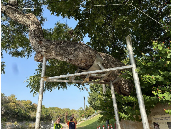
Image 4. Previously installed props used to support weight of the pecan's leaning stem.
