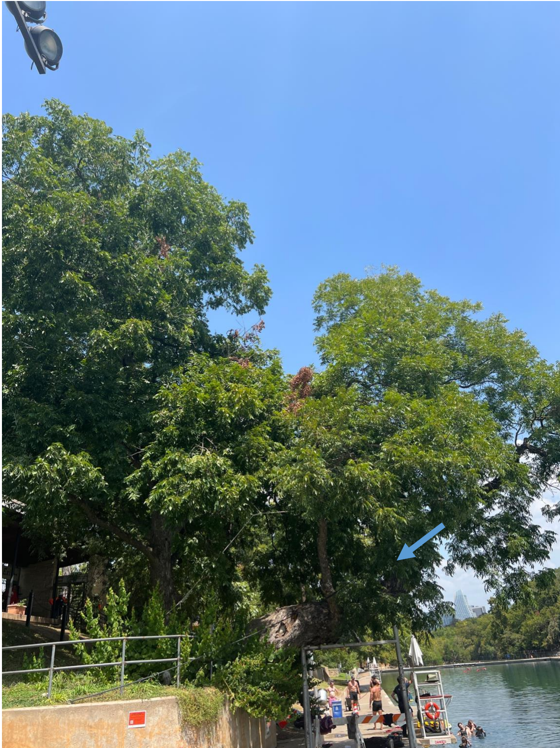
9: opposite view of target area and defect at second support point.
