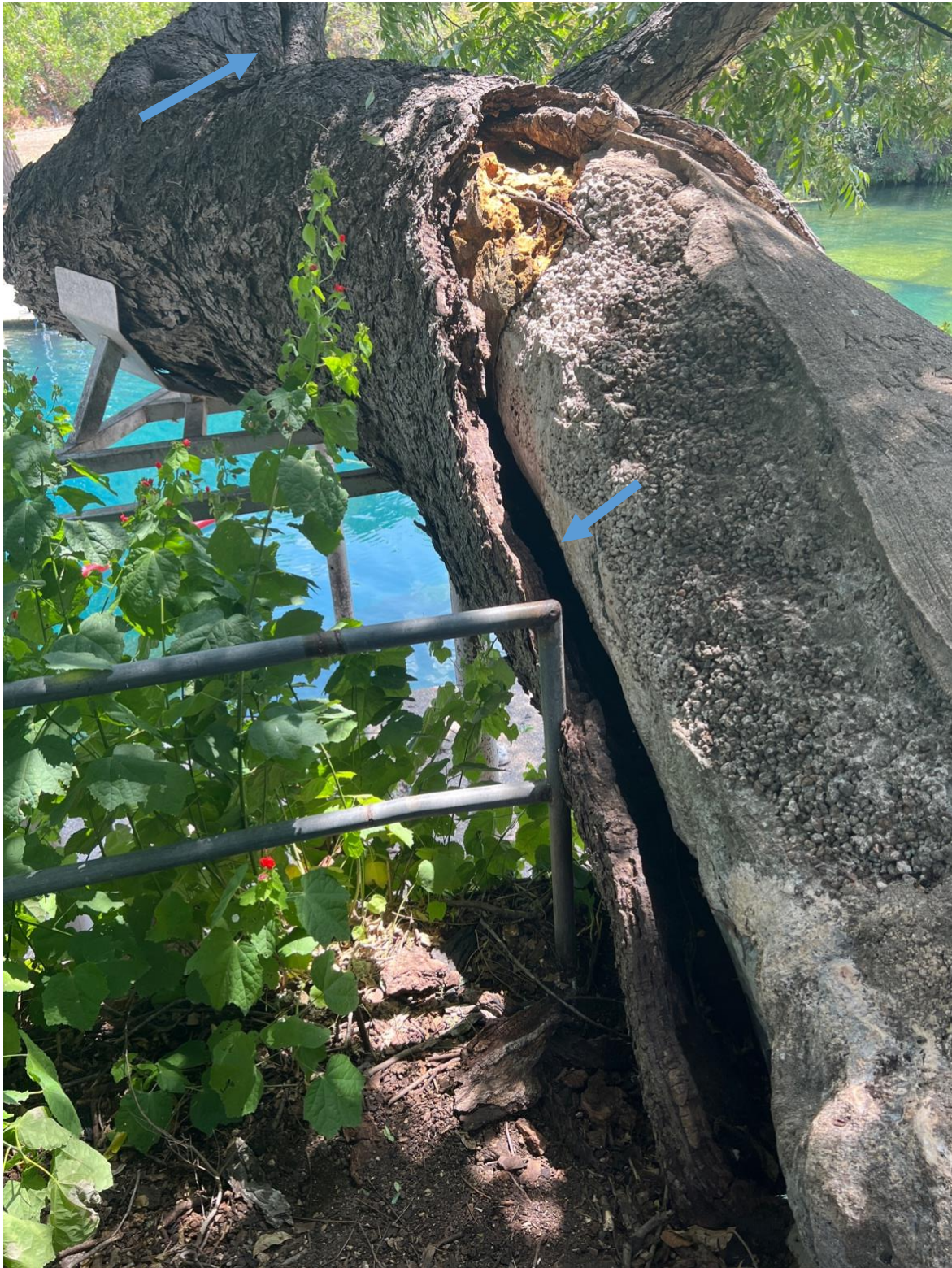
6: extend of heartwood loss, alternate view of defect at second support point.
