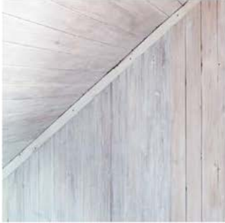
REFINISHED, REINSTALLED WOOD PANELING
