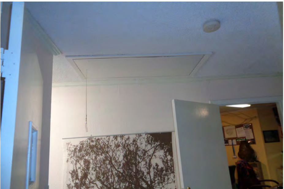
Sheffield Center Storage Space: Operation of the Sheffield Center is facilitated by the utilization of a mezzanine above the classrooms, accessible through this pull-down ladder.
