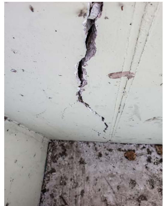
Structural cracks are observed in many concrete walls.
