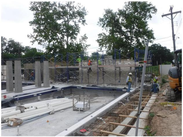
Limestone facing installation at Bathhouse in background. Shade structure columns in foreground. Note decking form work being prepared for concrete pour.
