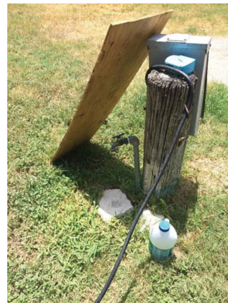
RV Water Spigot and Electrical Hookup
