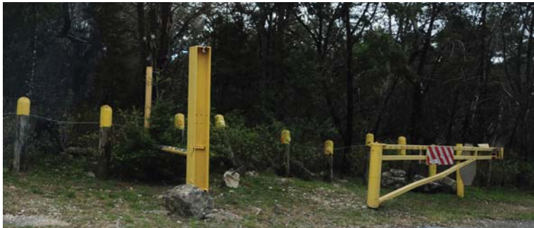
Control Gate at City Park Road and Pearce Road South
