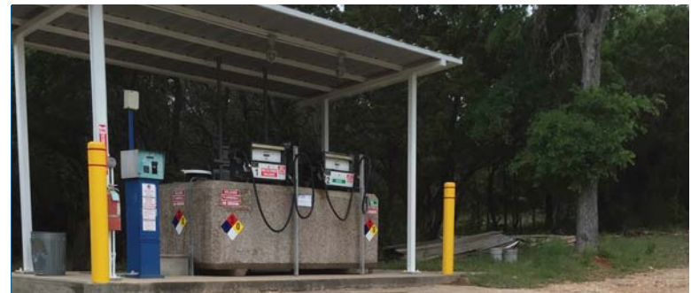
Fueling Station for Park Maintenance Vehicles
