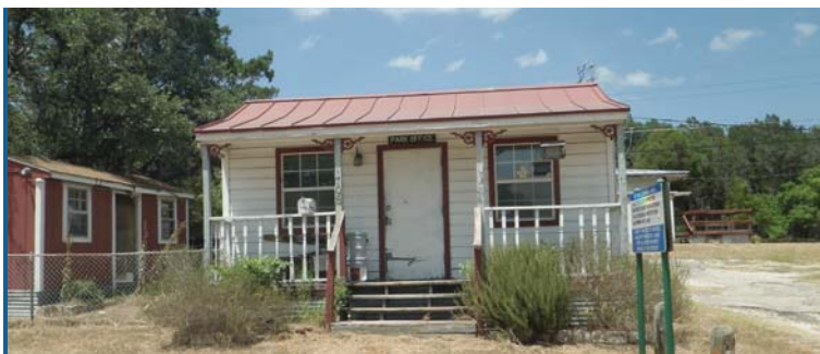
Park Maintenance Building
