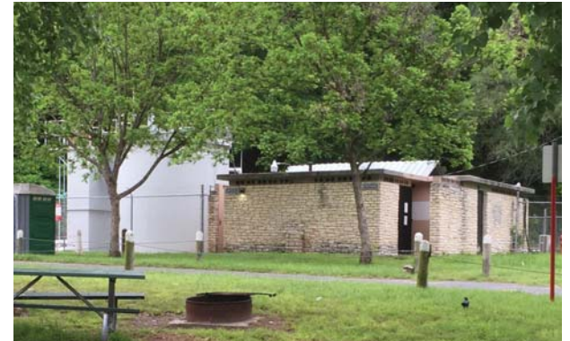
Campsite Restroom Building
