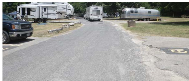
Pavement within the RV Area
