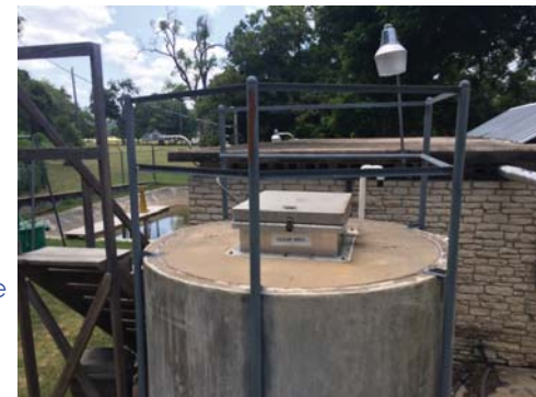
Clear well with treated water
