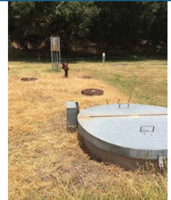
Wastewater Treatment Tank leading to Disposal Field
