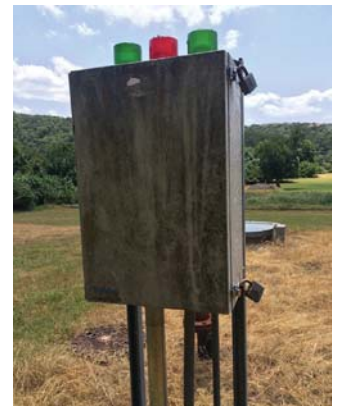
Wastewater Treatment Tank control panel
