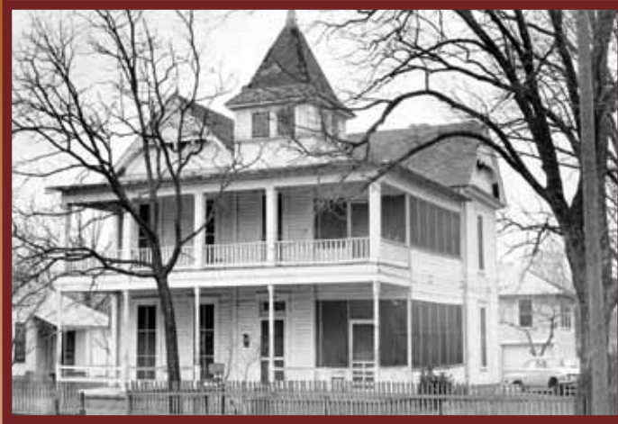
1804 E. Cesar Chavez St. (demolished)
