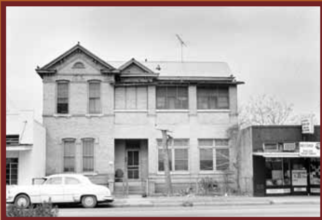
1112 E. Cesar Chavez St. (demolished)
