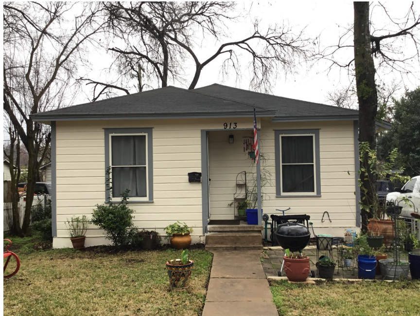
Figure 25. Example of a hipped-roof Minimal Traditional-style residence constructed in 1948 at 913 East 48 th Street (Survey ID 216435_01). Characteristics of the style include the small form, low-pitched and simple roof form with small eaves, small entry stoop, one type of cladding, and lack of decoration. Photo: CMEC.
