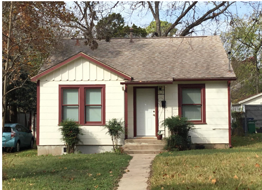
Figure 24. Example of a 1946 Minimal Traditional residence with a gable-and-wing roof at 3510 Hollywood Avenue (Survey ID 209163_01). Note the small and compact form, shallow eaves, small stoop with a simple prefabricated
