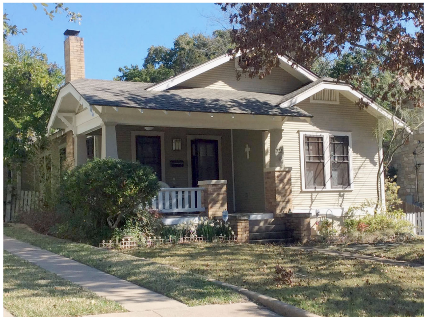
Figure 19. Typical example of an early 1920s Craftsman bungalow at 722 Sparks Ave (Survey ID 208723_01). The building features two front-facing clipped gables, a partial-width porch with tapered supports on brick piers, brackets and exposed rafter tails, a prominent brick chimney, and decorative window screens. Photo: CMEC.
