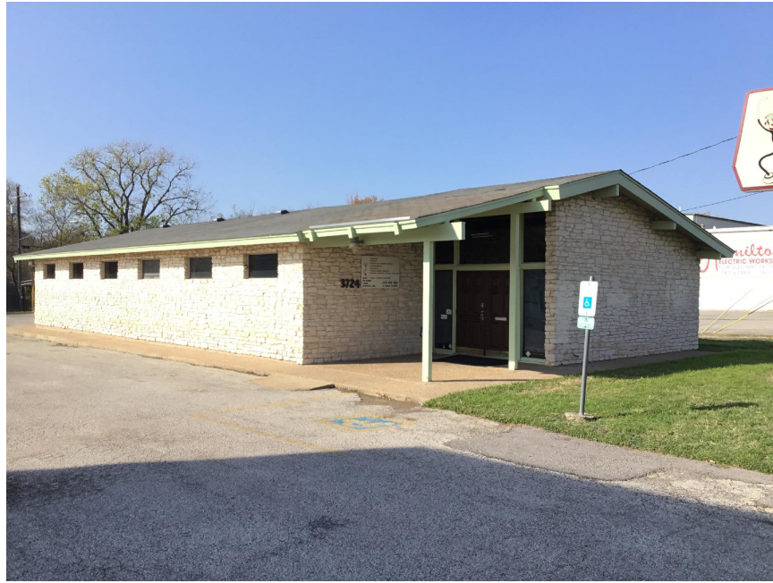
Figure 35. Post-war Modern-style commercial building at 3724 Airport Boulevard constructed in 1968 (Survey ID 207581_01). The post-and-beam construction typical of the style is evident in the exposed purlins and rafter tails near the primary entrance. Photo: CMEC.
