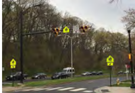
Pedestrian hybrid beacon on a divided roadway
