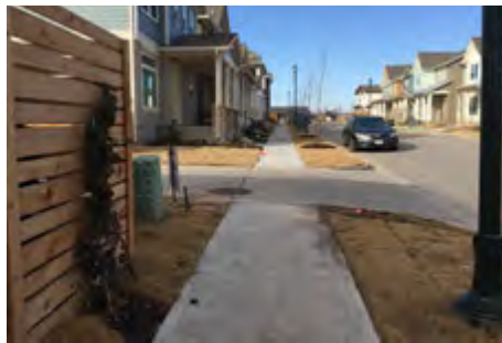
New sidewalk remains level across driveway
