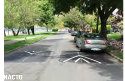
Speed cushions installed on hills may include a cut for downhill bicyclists
