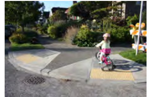
Each corner should have two curb ramps, one for each crossing
