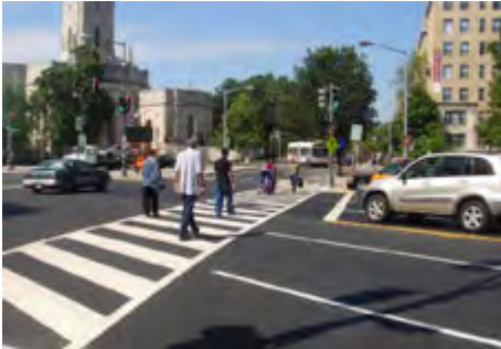
Marked crosswalk at an intersection
