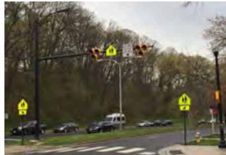
Pedestrian hybrid beacon on a divided roadway
