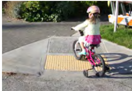
A sidewalk retrofitted with a curb ramp and a tactile warning strip
