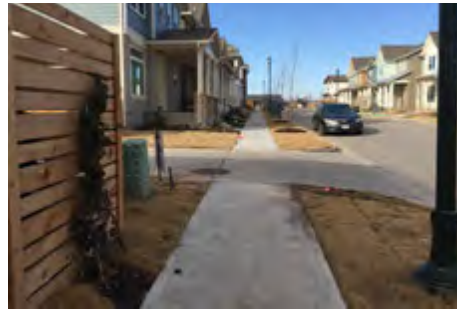
New sidewalk remains level across driveway
