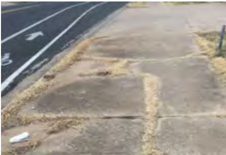
Severe cracking creates uneven and hazardous walking surfaces
