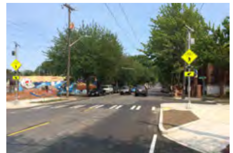
RRFB at a neighborhood bikeway crossing
