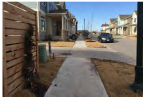
New sidewalk remains level across driveway
