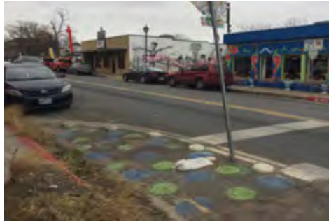
Easy-to-install materials such as paint, turtle bumps, and flex posts may be used to create curb extensions
