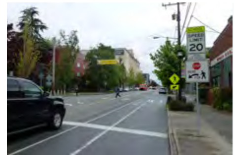
Advanced stop bars increase visibility of people crossing the street
