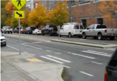
Mid-block curb extension
