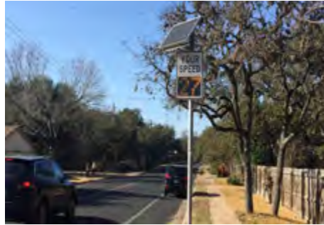
Solar-powered speed radar sign
