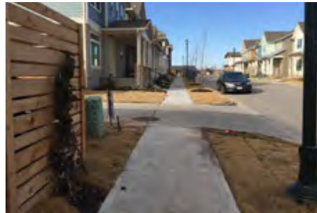
New sidewalk remains level across driveway
