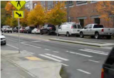
Mid-block curb extension
