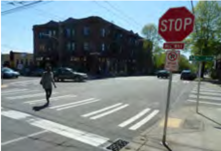
Stop sign with stop line at an all-way stop
