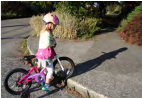
Curbs limit universal accessibility and are barriers for transitioning from the sidewalk to the street
