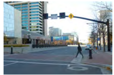
Pedestrian hybrid beacon on a downtown street
