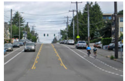
Center turn lane narrowed to provide space for bike lanes
