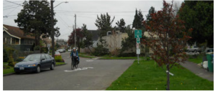
Signage and pavement markings help direct Neighborhood Bikeway users to destinations
