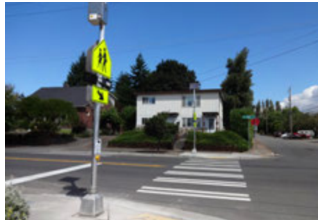
RRFB with push button at a school crosswalk
