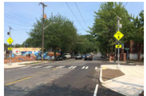
RRFB at a neighborhood bikeway crossing
