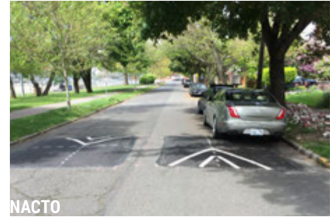
Speed cushions installed on hills may include a cut for downhill bicyclists
