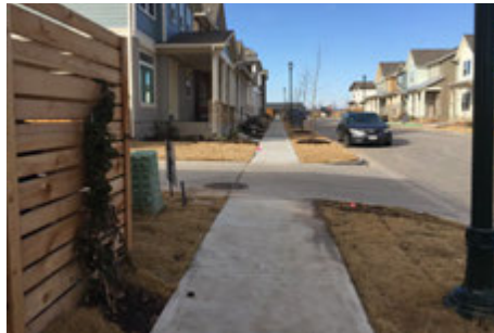
New sidewalk remains level across driveway
