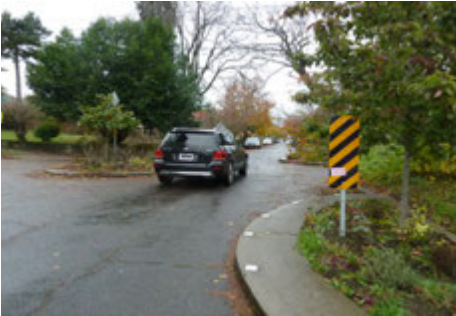
The horizontal deflection of chicanes and traffic circles force drivers to slow down
