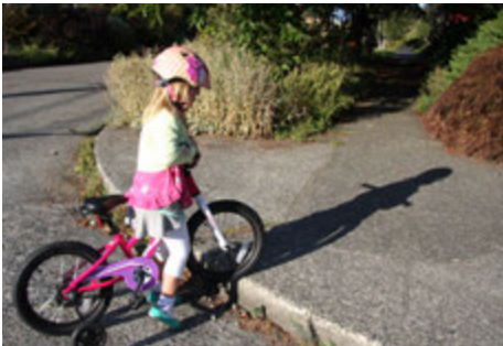
Curbs limit universal accessibility and are barriers for transitioning from the sidewalk to the street
