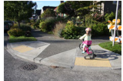
Each corner should have two curb ramps, one for each crossing
