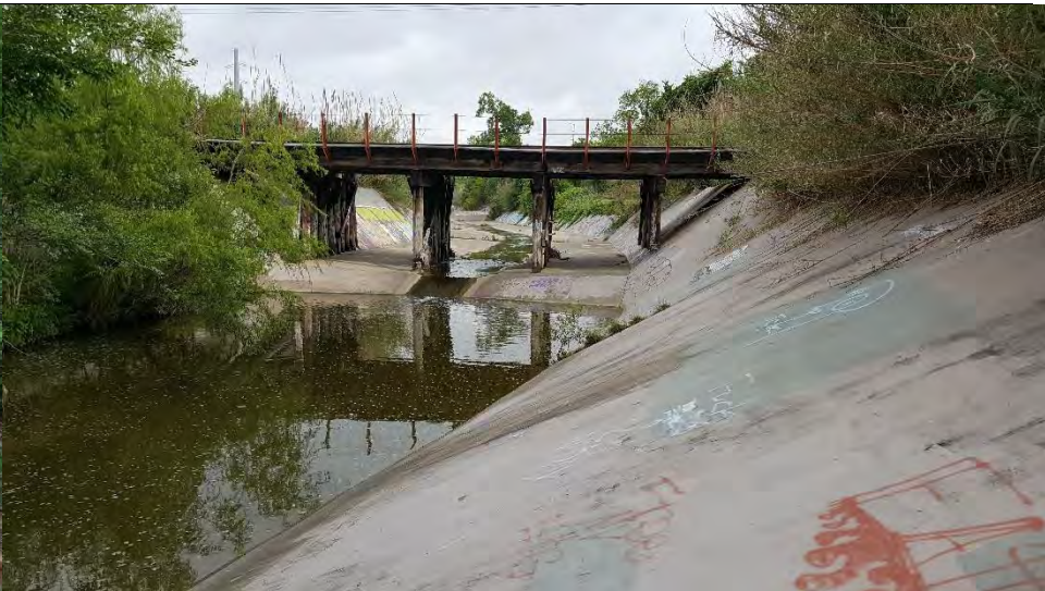
6. Looking North: Railroad crossing the Tannehill Branch Creek. Concrete lined open channel. The rail road bridge looks pretty old. There is an existing beaten pathway connecting this area which shows that the students cross the track underneath the bridge.
