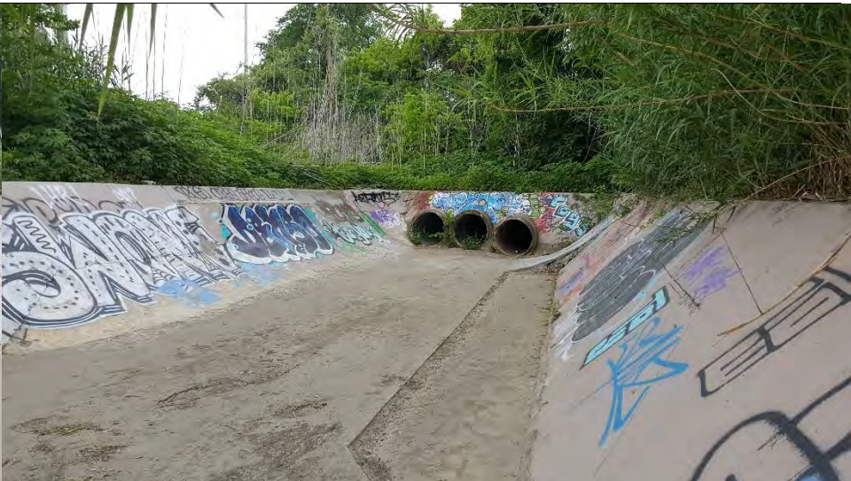
14. Tannehill branch - Crossing 2 – 3ft Diameter three RCP.
