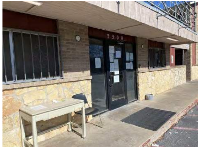
Leasing office exterior
