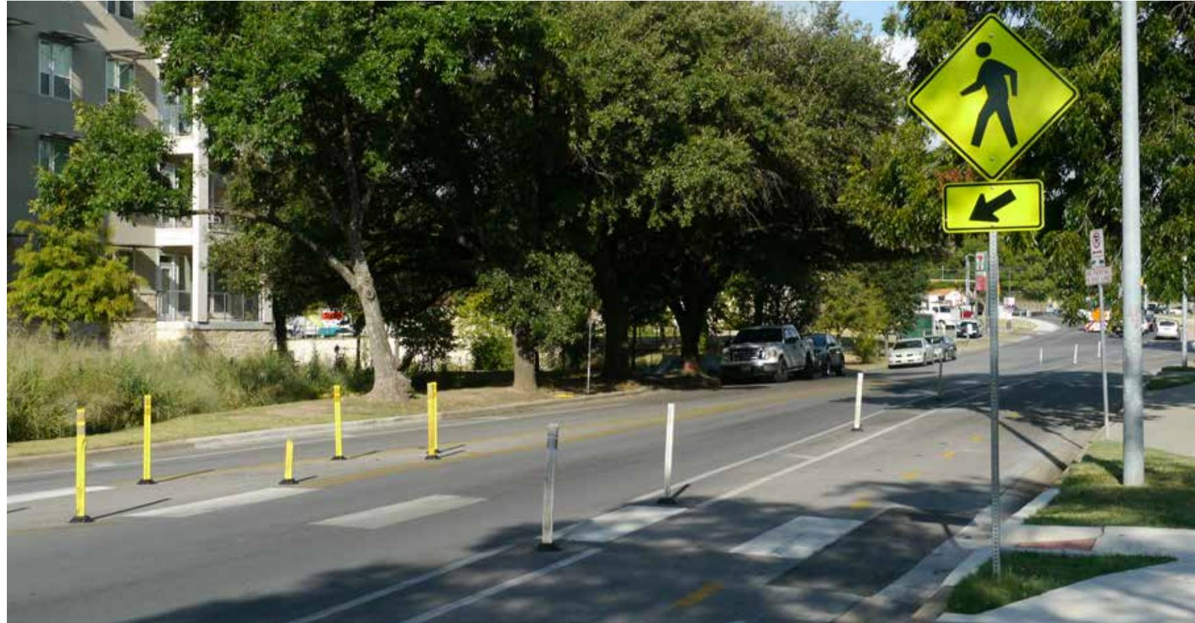
A pedestrian median island helps to encourage yielding by drivers and makes it easier for a person crossing the street to focus on one lane of oncoming traffic at a time.
