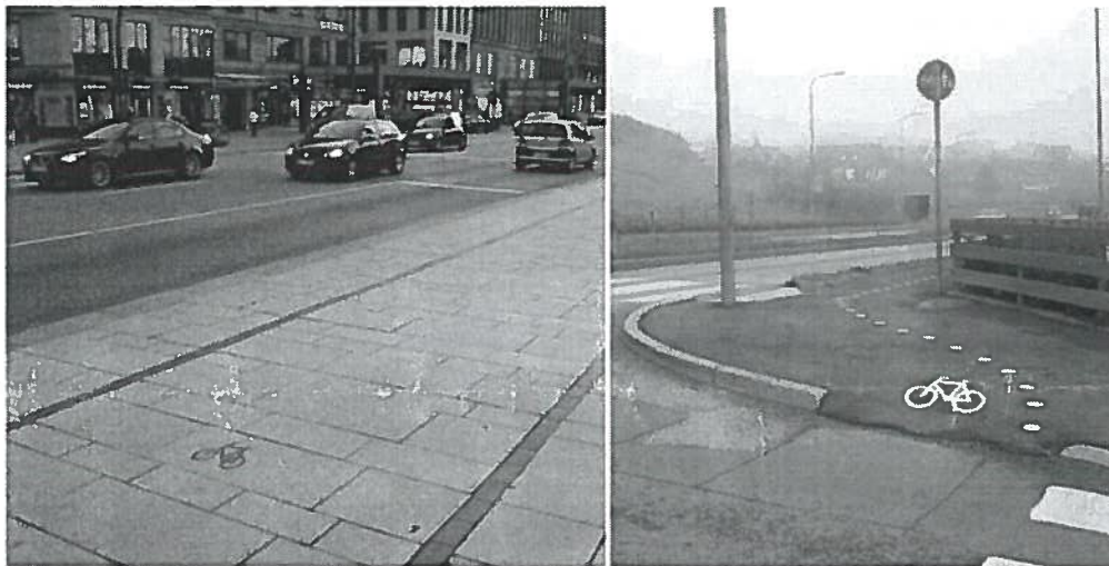
Figure 5.9 Left: Bicycle track (barely) marked on the sidewalk (Germany) Right: Bicycle track marked on the sidewalk (Faroe Islands)
