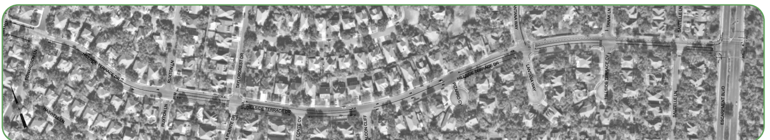
For a detailed drawing on changes on Hillside Terrace Drive, please visit the project webpage .
