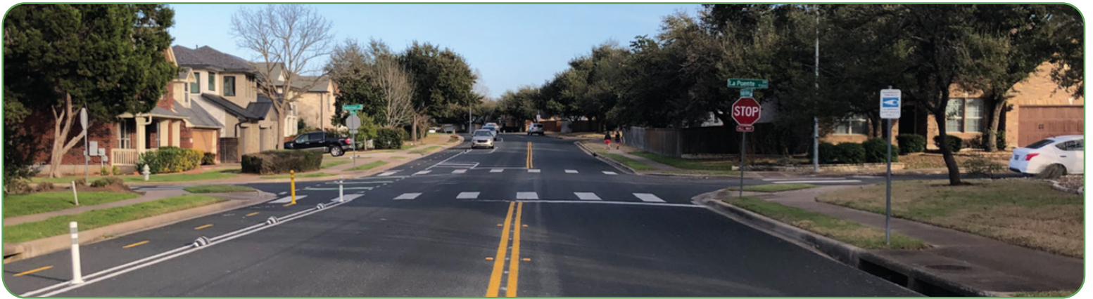
Existing conditions on Hillside Terrace Drive
