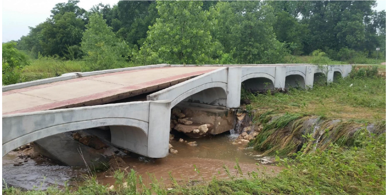
Figure 3-1: Severe flooding in 2015 damaged and later destroyed a trail bridge in Roy G. Guerrero Park. Replacing the bridge was delayed for several years due to ongoing erosion challenges. Credit: Austin Parks And Recreation Department
