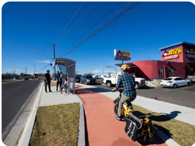
Floating Bus Stop on Stassney Lane at South 1st Street Source: City of Austin
