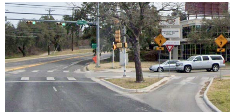
“Smart right” turn on N Lamar Boulevard at W 29th Street, Austin, TX Source: Google Street View
