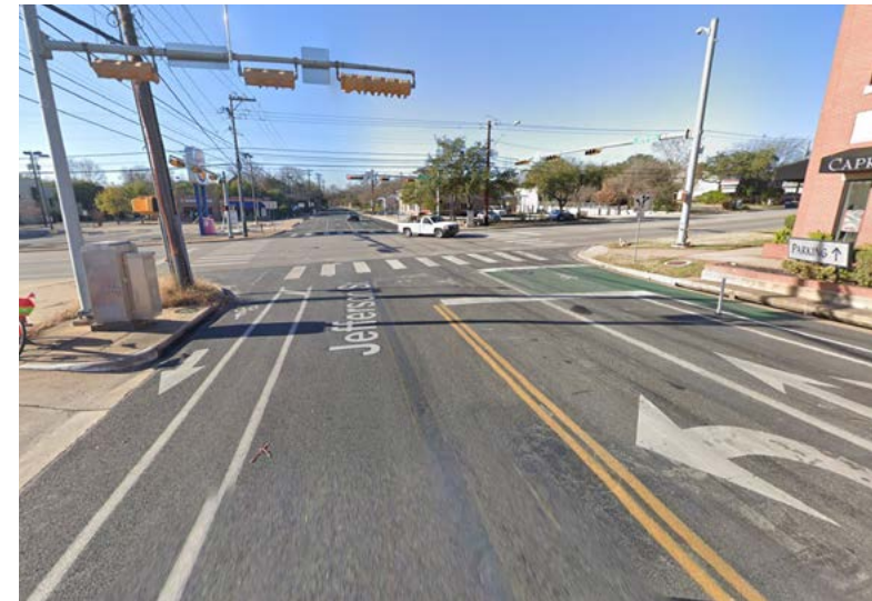
Right turn pocket on 7th Street at I-35 (Austin, TX) separates right turning vehicles from through moving buses
