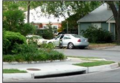
1. Inlets and curbs capture rainwater.
