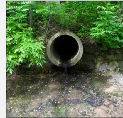
3. Rainwater is released into a creek at the outfall. Sometimes it goes to a pond first.
