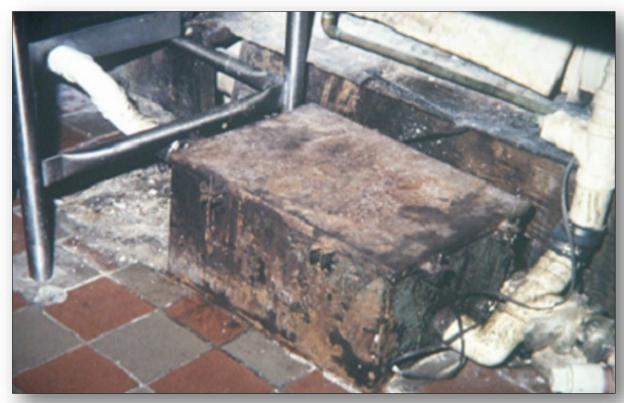
The under-counter grease traps like the one to the right are no longer approved.
