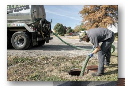
The FOG and solids must be removed regularly for the grease trap to work properly.
