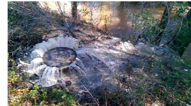
Fuente de la imagen: Grease Blockage causes another Alpine Utilities sewage overflow
