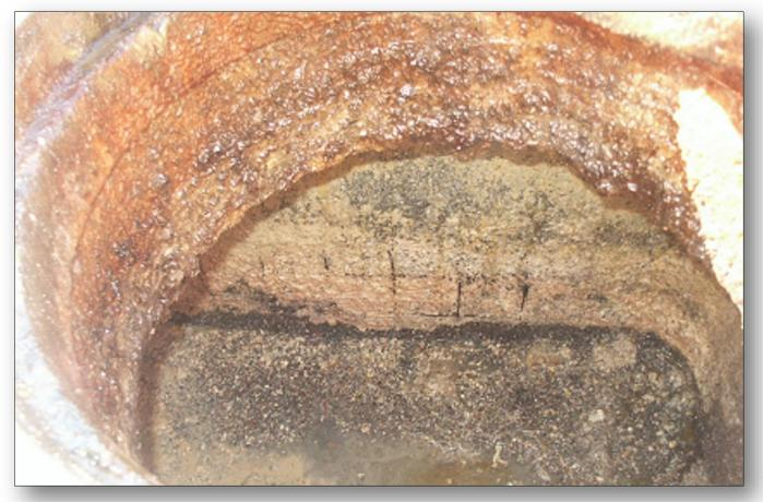
Notice the black lines on the tank wall of the trap shown above. This is exposed wire rebar.
