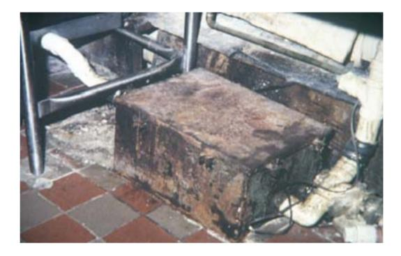
A trap that is too large may be just as problematic. Oversized traps may become stagnant, causing odor problems and/or corrosive conditions that drastically shorten the trap's useful life. The design of the trap is as important as its size. Note the short distance between the inlet and the outlet. This old style cylindrical trap is no longer approved for installation because of its poor performance.
