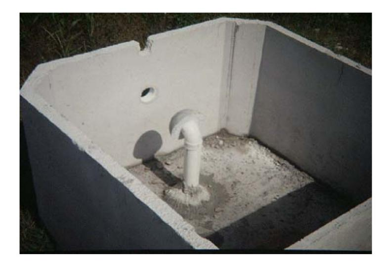
Here, the baffle wall and piping can be seen. Proper baffling insures that the flow is evenly spread throughout the tank.
