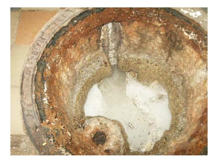
The undercounter grease traps like this one are no longer approved. The smallest sized grease trap approved for installation today is 100 gallons.
