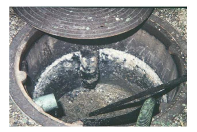
Note the flow diverter on inlet side of this new installation. This helps to eliminate channeling effects or "short circuiting."
