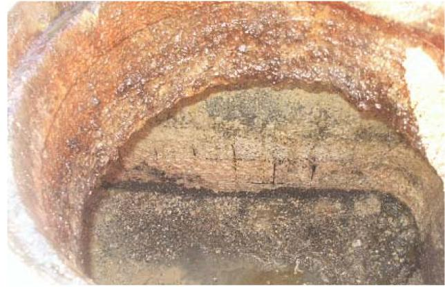
These acids are very destructive and over time can cause baffles, piping, and tank walls to simply crumble apart. Notice the black lines on tank wall of the trap shown above. This is exposed wire rebar. Grease traps are very expensive to install and/or replace. Making sure they are cleaned and pumped out on a regular schedule is very important.
